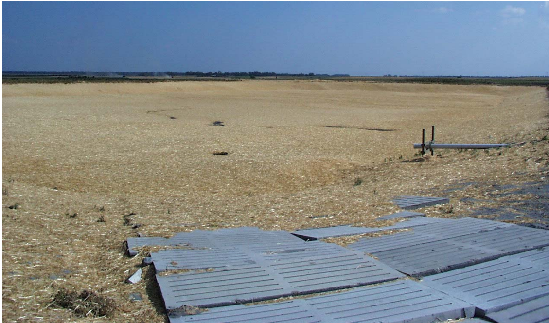
Figure 2. Permeable Straw Cover Installed on an Earthen Manure Storage Structure
