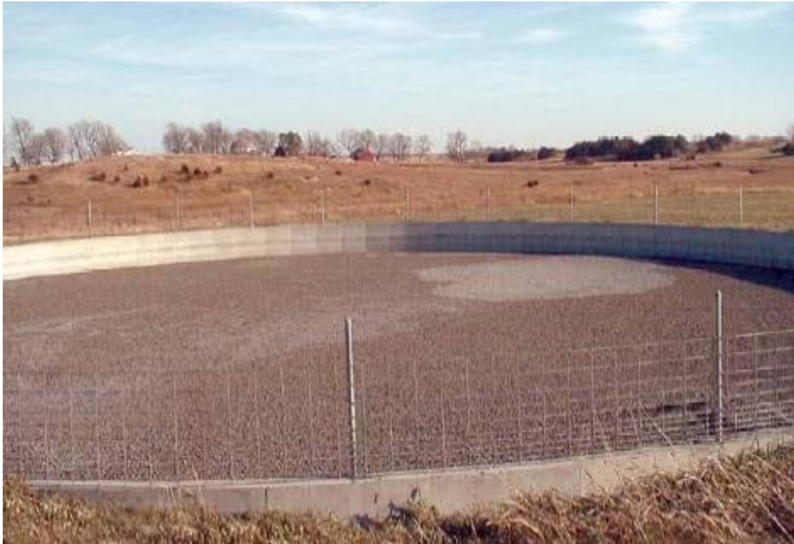
Figure 3. LECA Cover on A Concrete Swine Manure Storage Tank
