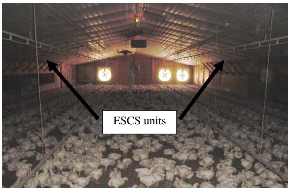
FIGURE 1. Electrostatic space charge unit assembly within a broiler house.
