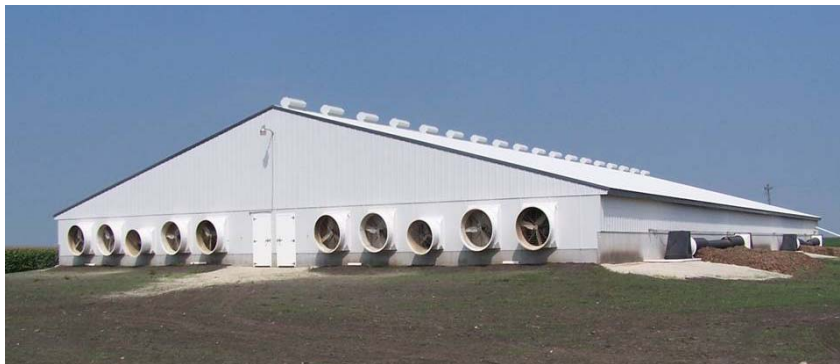
Figure 1. 2400 head, deep-pit, pig finishing barn with biofilter treated air from pit fans
