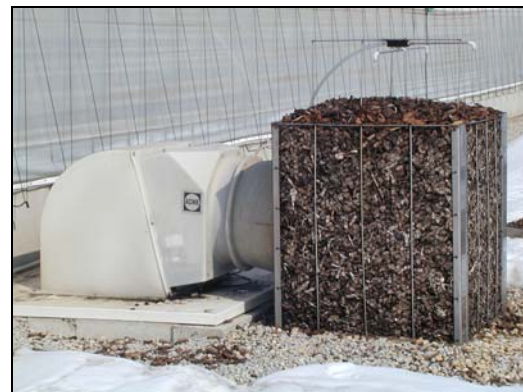
Figure 2. Mature odor cell with hydrator
