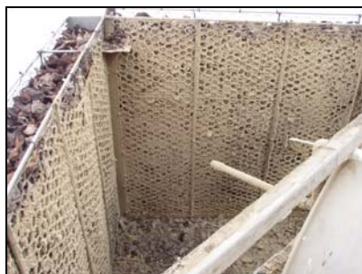
Figure 3. Non-hydrated filter after 4 months of operation.
