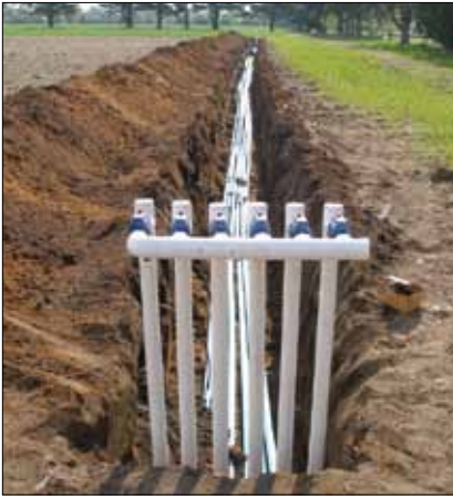
Sub-surface irrigation being installed in 2007 for research.
