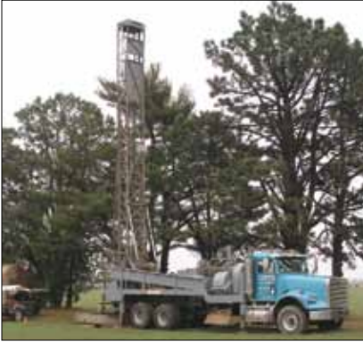
Well-drilling equipment at the installation of sub-surface irrigation system.
