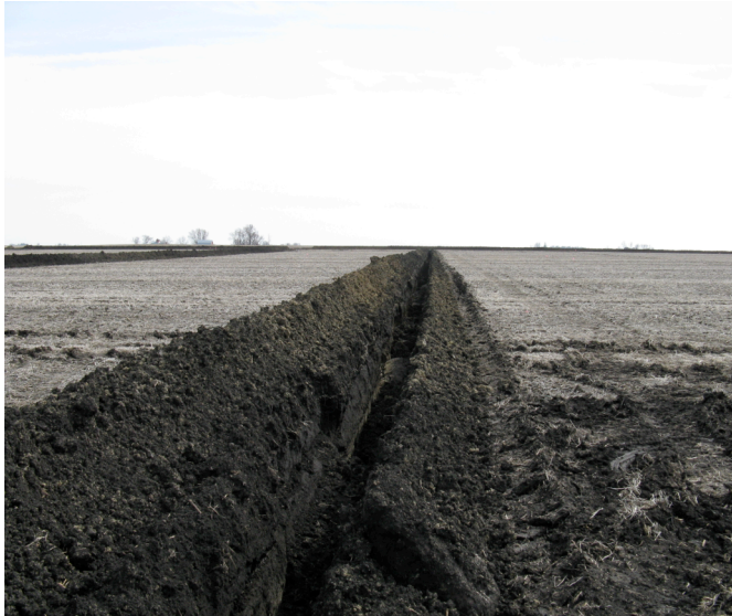
Figure 1. Picture of tile installation in Spring 2008.
