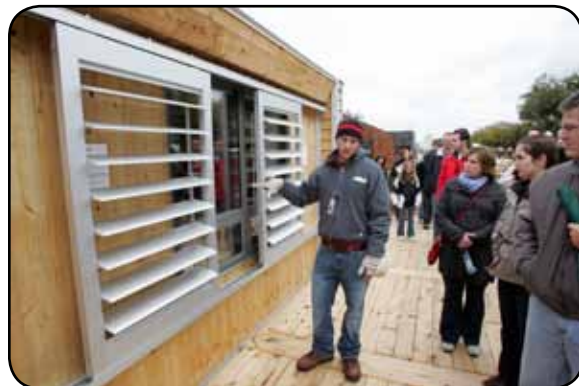
Stefano Paltera, US Dept. of Energy Solar Decathlon Iowa State student Thomas Dillman shows visitors the adjustable window louvers used to prevent direct heat gain.
